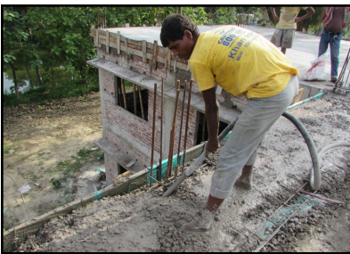
Use of vibrator to spread the mixture properly
