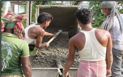
Unload Cement Mixture
