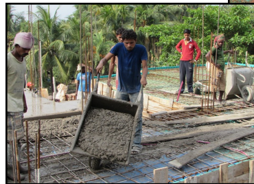
The Concrete Mixture is taken to the roof
